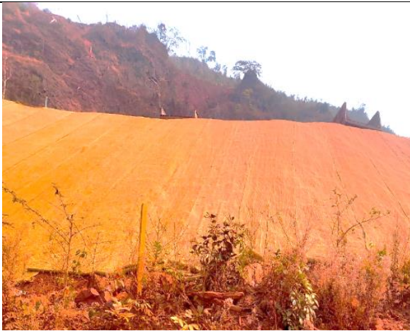
Coir mat application on dump slopes
